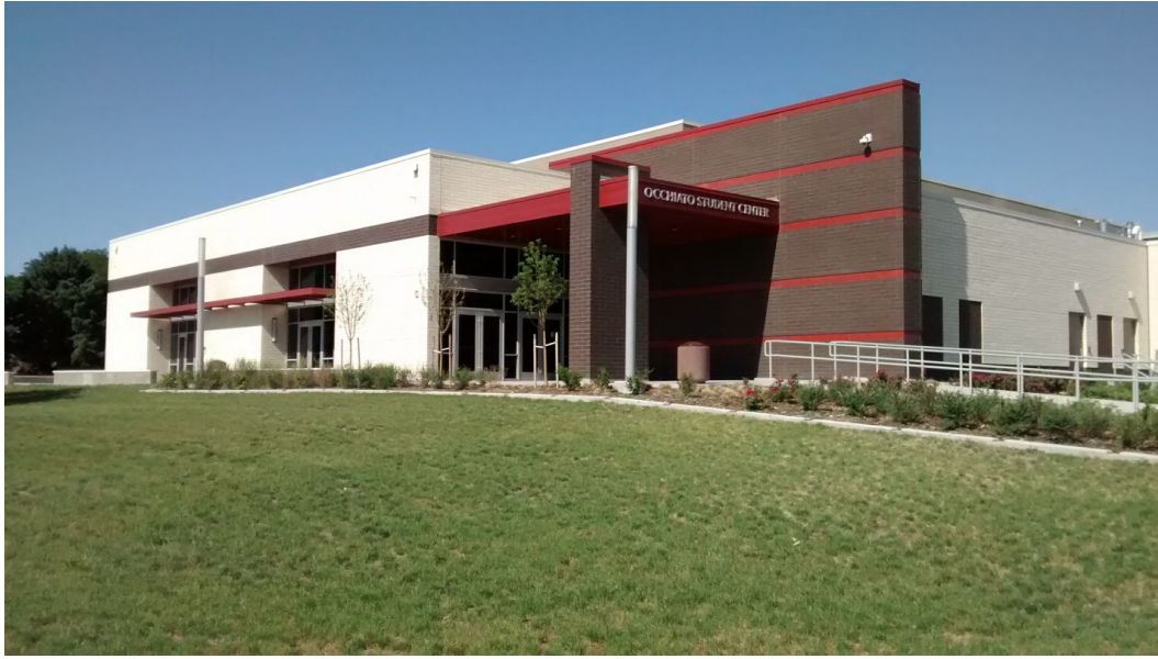
Occhiato Ballroom Entrance
